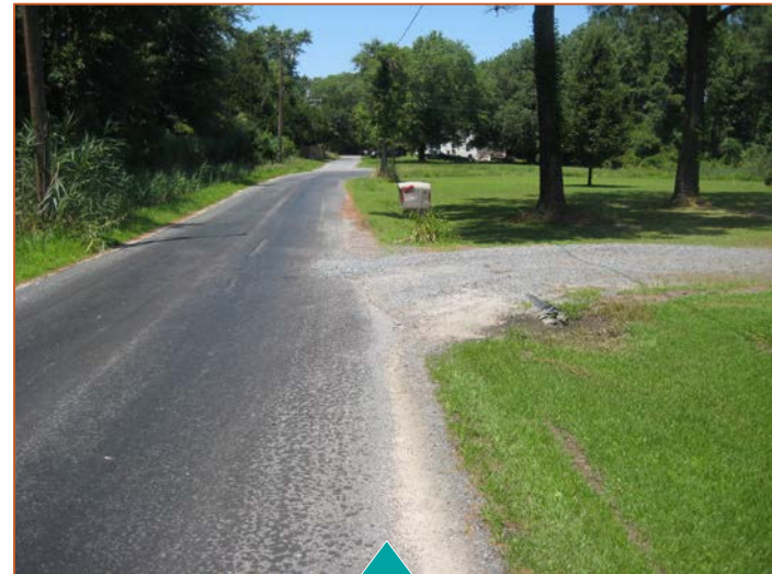
Hodson White Road Buried driveway HDPE culvert
