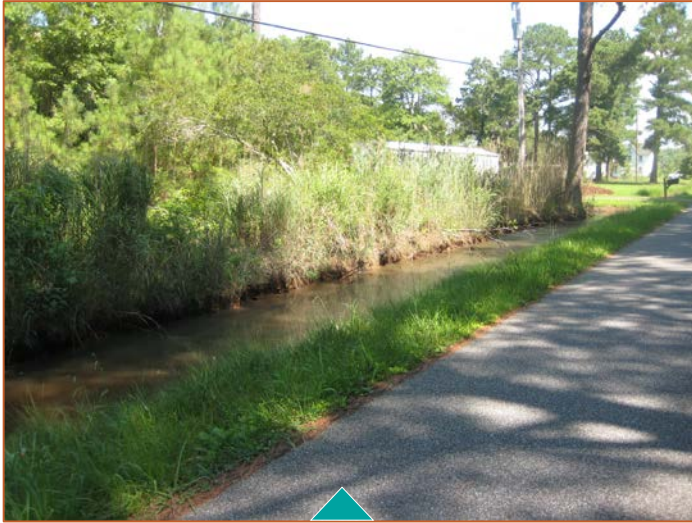
Champ Road Standing water (south of 10006 Champ Road)
