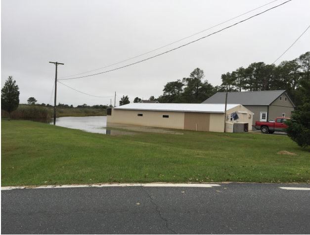
Top left: Flooding along Deal Island Rd. at Ford Rd. following a tropical storm during Fall 2016. Flooded shed is part of a commercial watermen business. Visible behind the shed is the Middle Creek marsh area (photo credit: M. Paolisso). Right: Abandoned property in Ballard Rd. neighborhood with marsh encroachment (photo credit: E. Van Dolah). Bottom left: Flooding during a storm on Ballard Rd. heading east towards Deal Island Road and John Wesley UMC. Middle Creek marsh is pictured on the right (photo credit: M. Paolisso).
