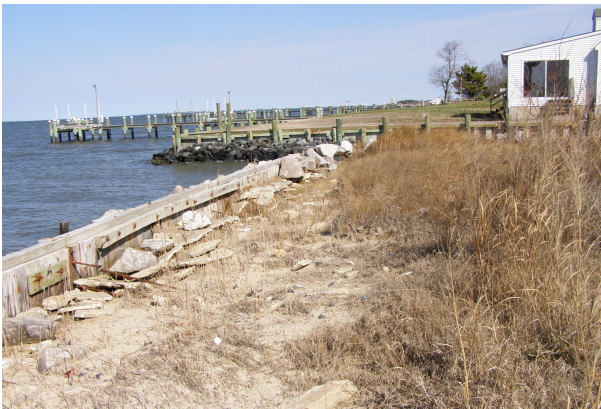
Top row: Deal Island shoreline beach erosion with ghost forest in background, photo taken from Crowell Rd.; Bottom row: damaged bulkhead and riprap on Tangier Sound shoreline with signs of erosion (Photo Credit: L. Collier).
