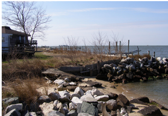
Top row: Deal Island shoreline beach erosion with ghost forest in background, photo taken from Crowell Rd.; Bottom row: damaged bulkhead and riprap on Tangier Sound shoreline with signs of erosion (Photo Credit: L. Collier).
