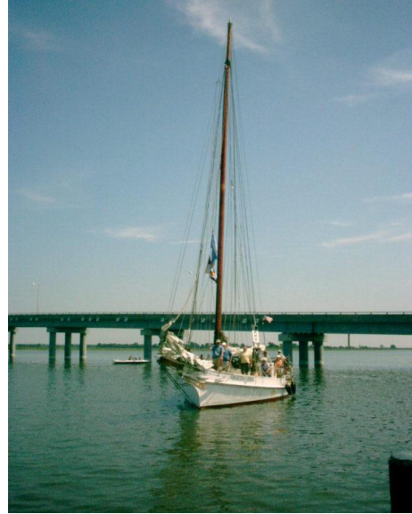
Deal Island Bridge 2003
